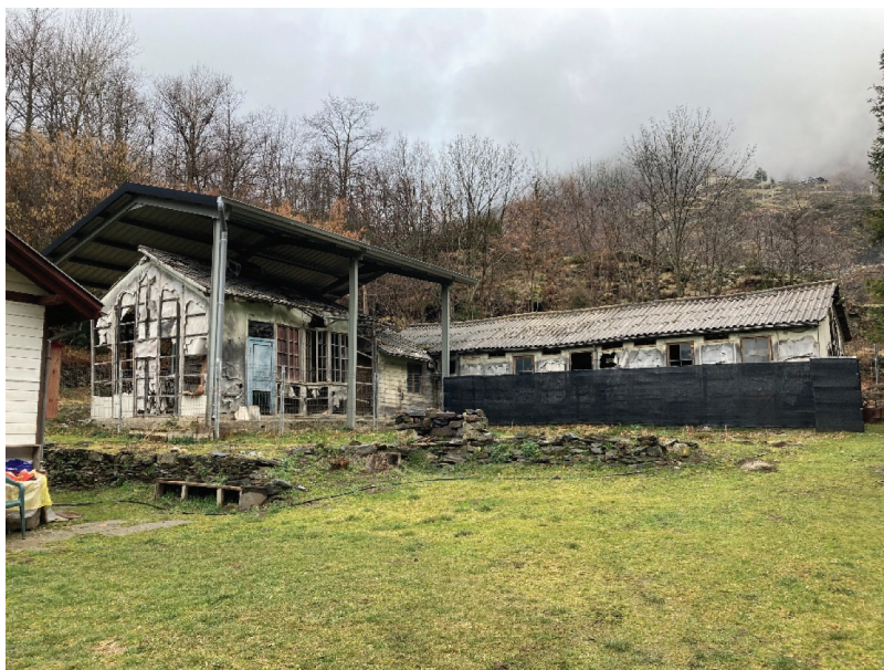
Figure 1. The cardboard hospital in March 2022. The surgical area can be seen in an advanced state of deterioration in the foreground, and the treatment wing is in the background in a better state of conservation. Source: Ana Pastor.
