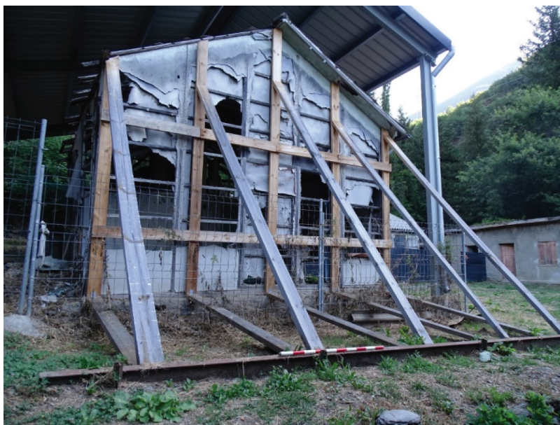
Figure 3. Props were installed to prevent the collapse of the surgical wing. August 2023. Source Ana Pastor.
