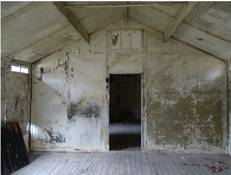
Figure 5. Treatment wing, middle stage after the initial cleaning works. May 2021. Source: Ana Pastor.
