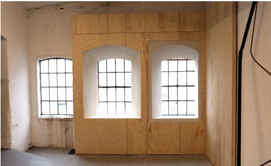
Fig. 7. Modules prototype 1 and wood-fiber back wall mockup
