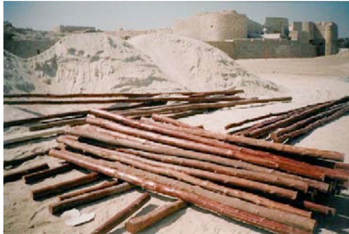
Traditional Structural Wood ( Danshil ) for Conservation/Restoration (October 2003)
