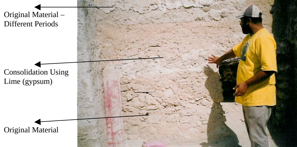
The Main Fortress ("Bahrain Fort"). Showing Original Wall (October 2003)
