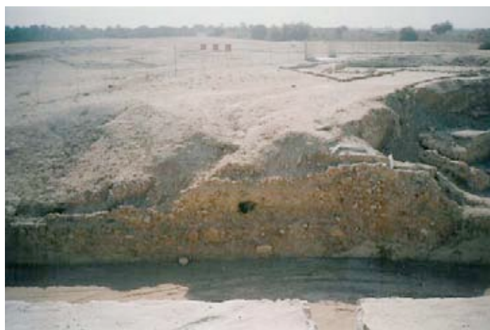
View of Moat (October 2003)
